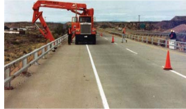
Under bridge unit may be necessary for proper bridge inspections access. (Note: inspectors on right of photo)
